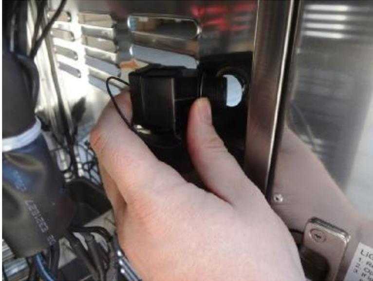
Mount the ignition module onto the grill in the same location that the old module was removed from.
