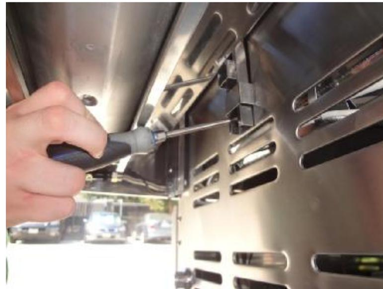
Secure the screw that goes into the center post of the side shelf, and then tighten the screws that mount on the left and right via the keyhole slots. Repeat steps 30 and 31 for the un-mounted side shelf on the opposite side.
