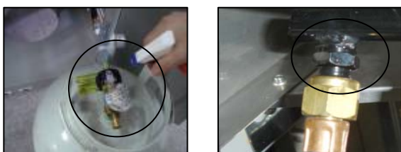
Gas Connection Leak Check
